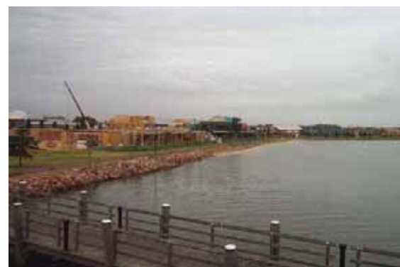
Housing construction in Newcastle
